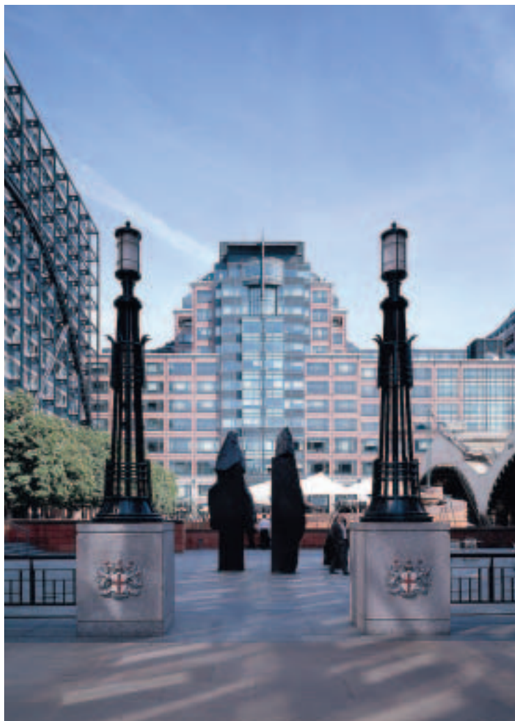
The Broadgate Centre
