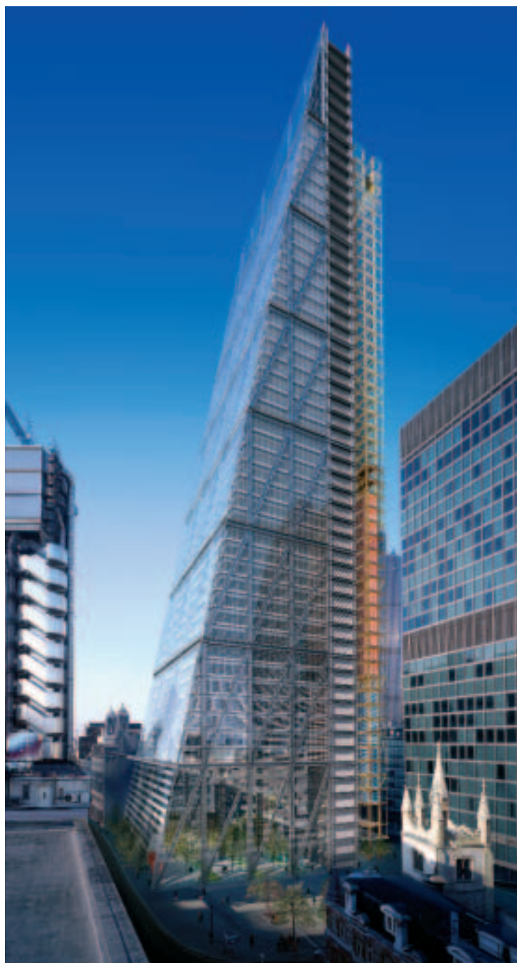
The Leadenhall Building viewed from the east. Computer generated image courtesy of Cityscape.
