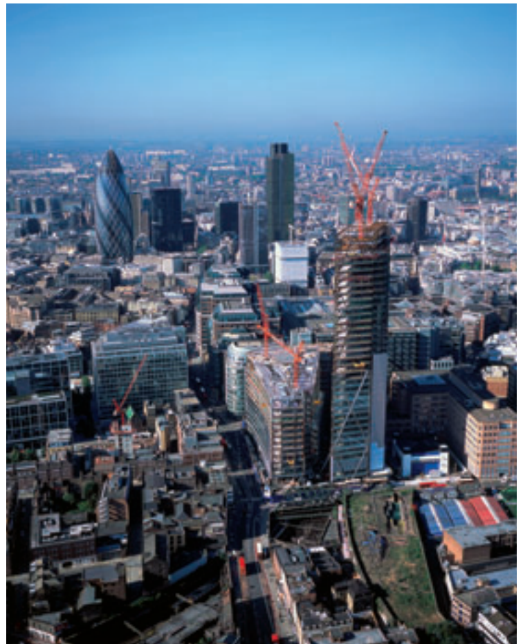
201 Bishopsgate and The Broadgate Tower, development under way
