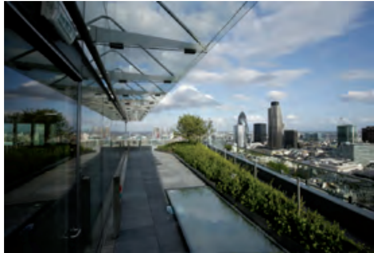
Green roof at Ropemaker
